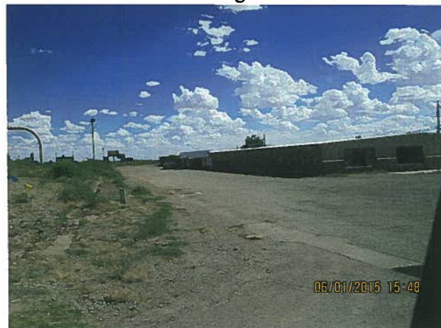
Vacant Commercial Building
