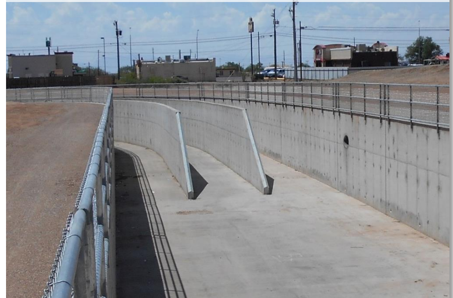
Rectangular Channel with Splitter Walls
