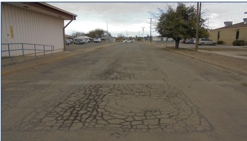
Subject property seen viewing in an easterly direction from the mid-portion of the property
