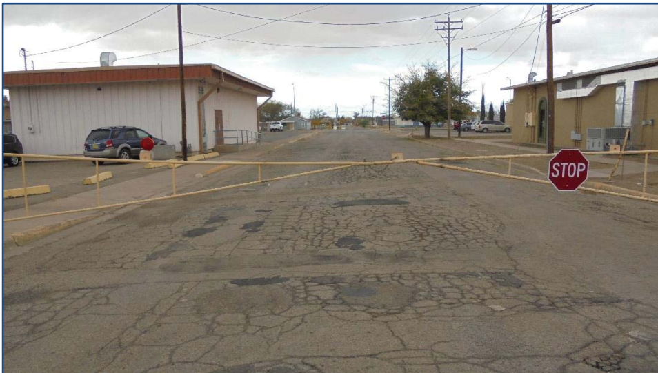
Subject property seen viewing in a westerly direction from near its east property boundary at the intersection of 13 th Street and Alaska Avenue
