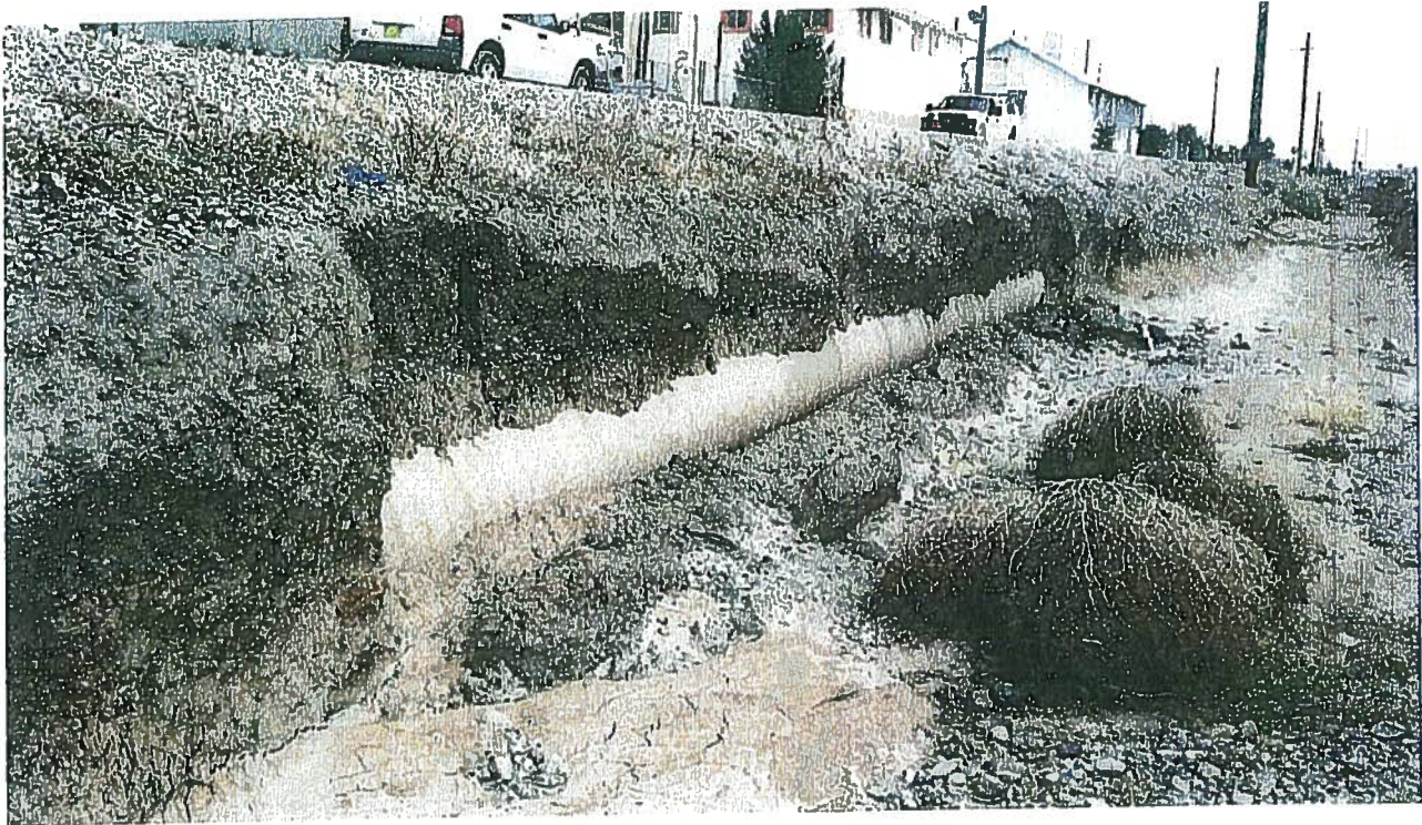
Photo 1. Existing 22-inch RCP
