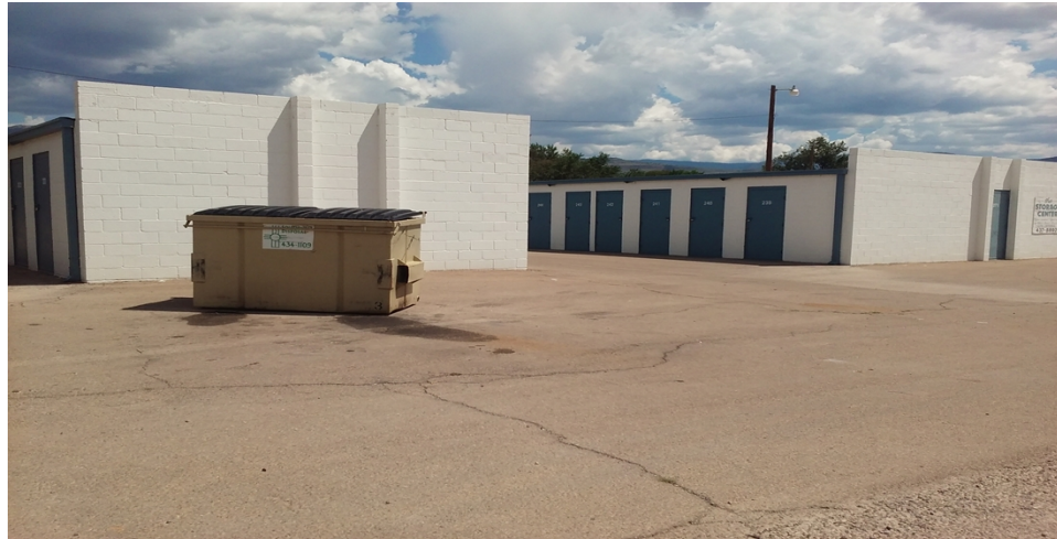
South - Storage Unit Facility – The Storage Center - M-1 (Light Industrial)
