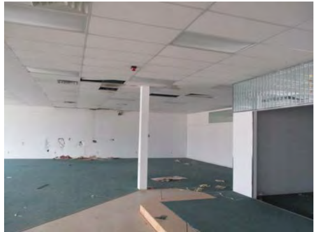
INTERIOR VIEW (NORTH BUILDING)
