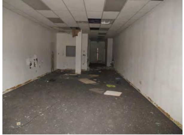
INTERIOR VIEW (SOUTH BUILDING)
