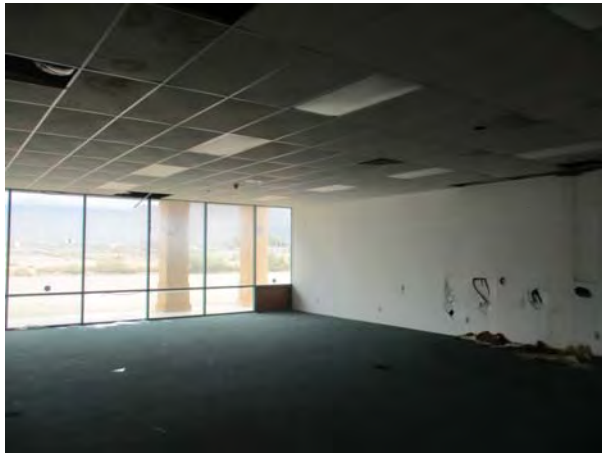
INTERIOR VIEW (NORTH BUILDING)
