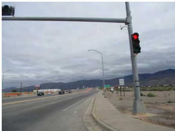
VIEW LOOKING EAST ALONG HIGHWAY 70
