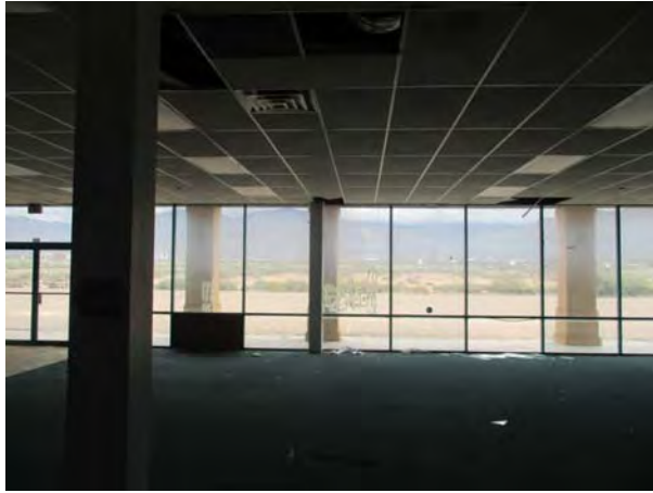
INTERIOR VIEW (NORTH BUILDING)
