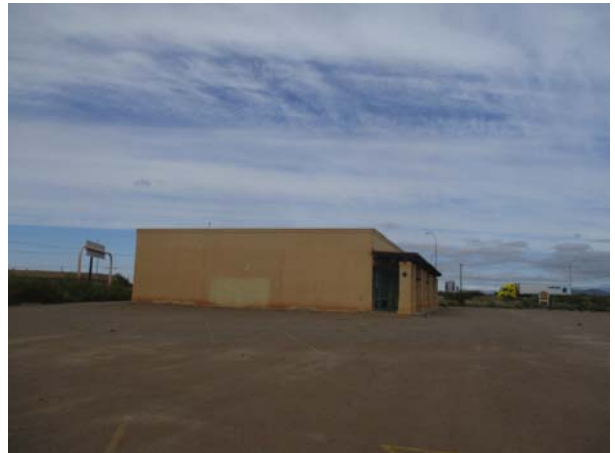
EXTERIOR VIEW (NORTH BUILDING)
