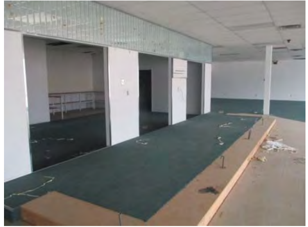
INTERIOR VIEW (NORTH BUILDING)
