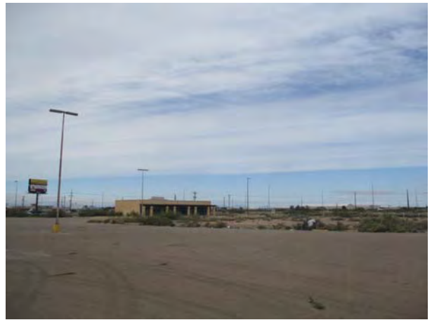
EXTERIOR VIEW (NORTH BUILDING)
