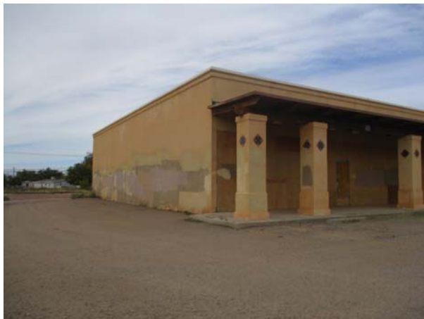
EXTERIOR VIEW (SOUTH BUILDING)
