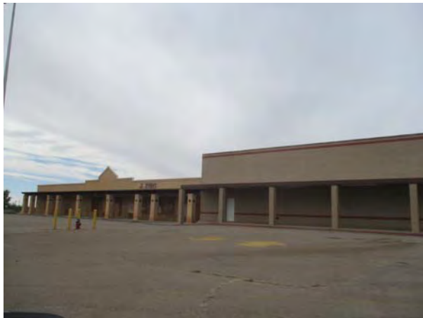
EXTERIOR VIEW (SOUTH BUILDING)
