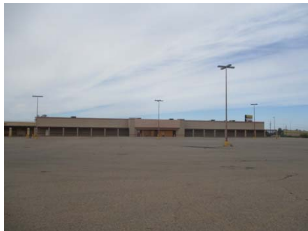
EXTERIOR VIEW (MAIN BUILDING)
