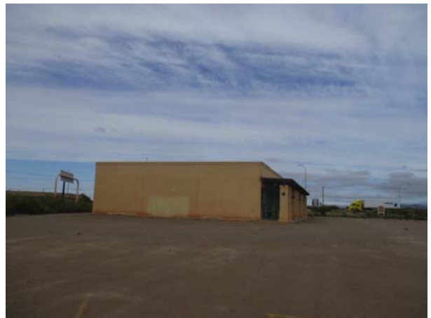
EXTERIOR VIEW (NORTH BUILDING)
