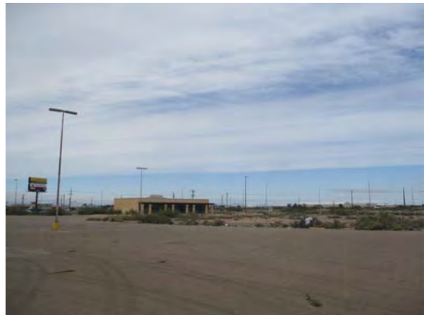
EXTERIOR VIEW (NORTH BUILDING)
