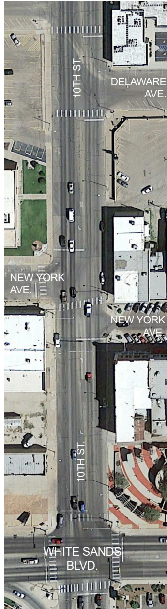
Aerial showing 10th Street from White Sands Boulevard to Delaware Avenue.
