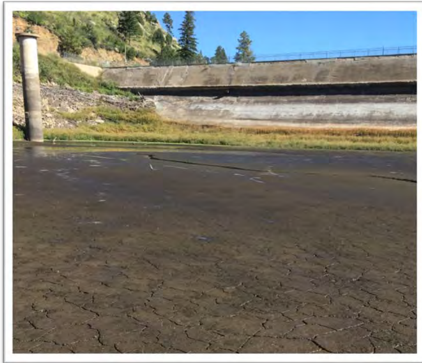
Saturated Debris after storm event
