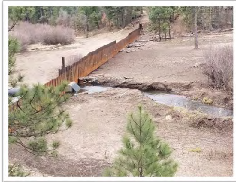
Coffer Dam Performing under normal conditions
