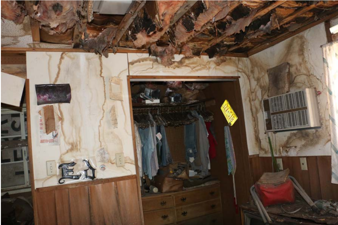
Photo #204 southeast corner room
