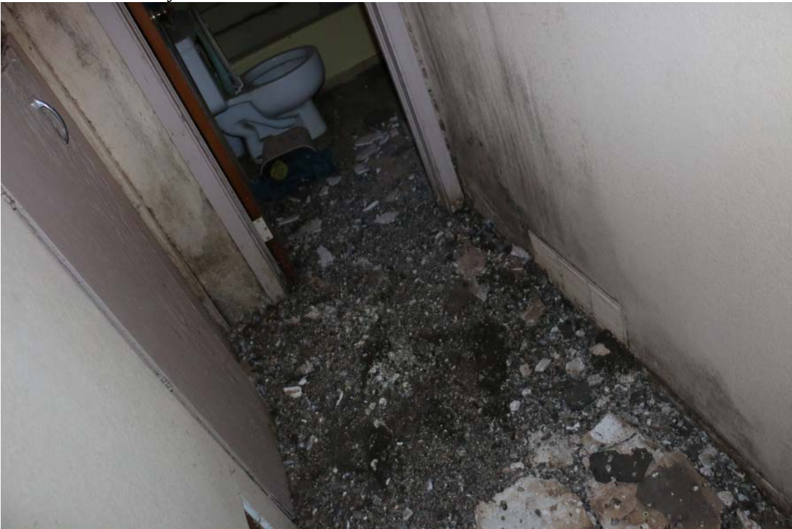
Photo #145 hallway to bathroom
