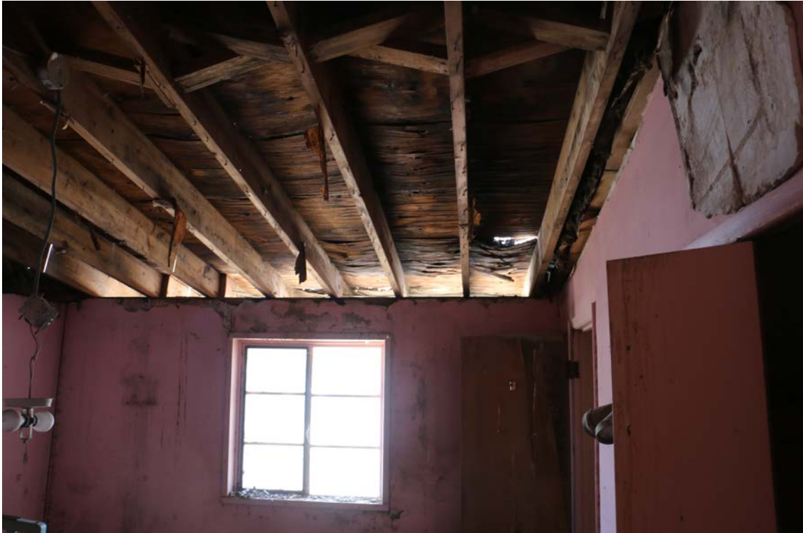
Photo #161 southside bedroom
