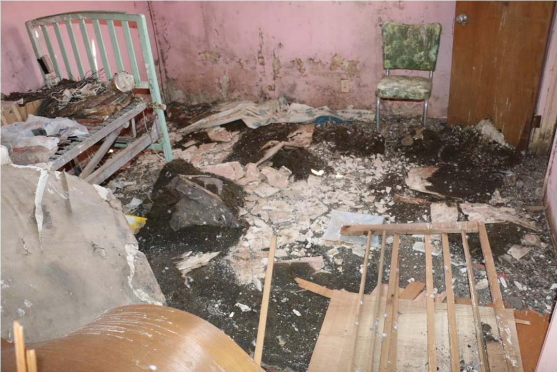
Photo #164 southside bedroom
