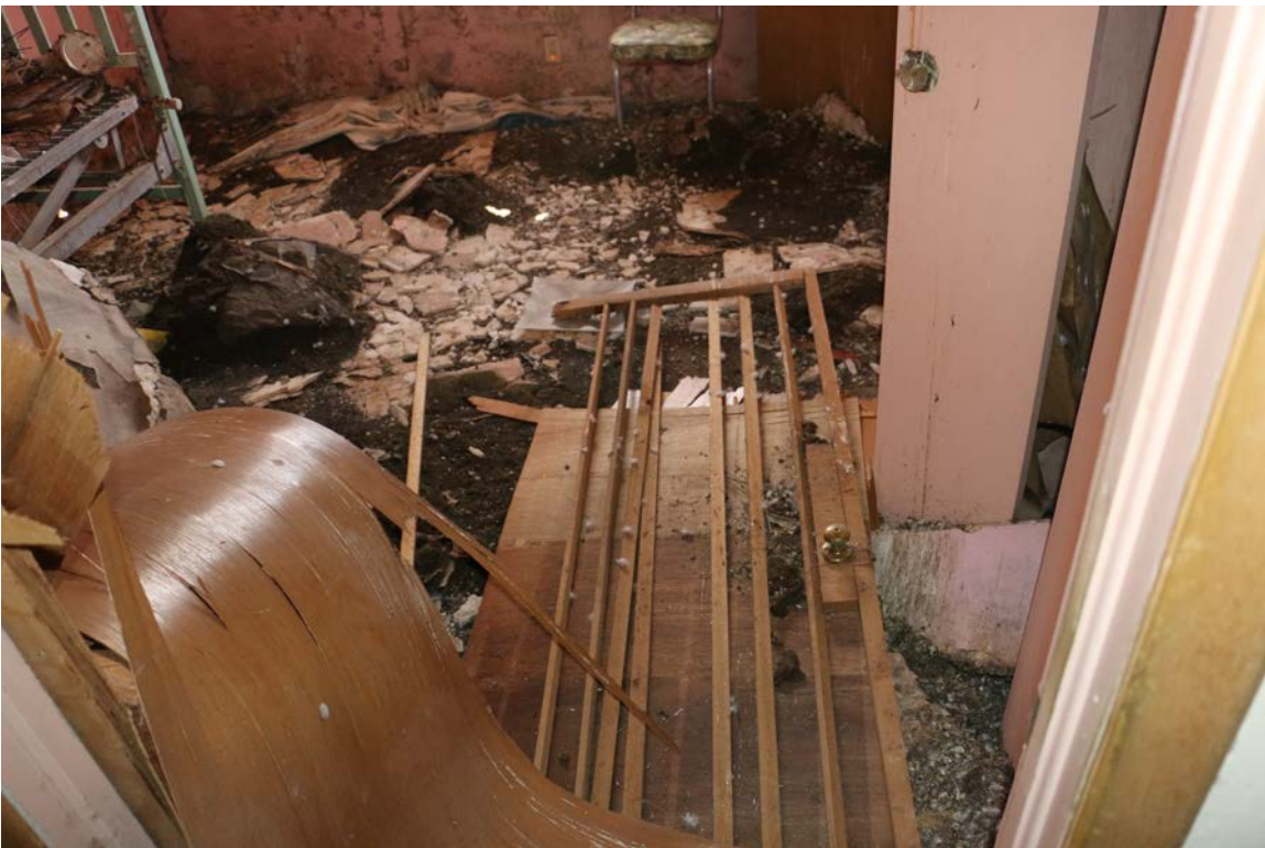
Photo #212 Southside bedroom
