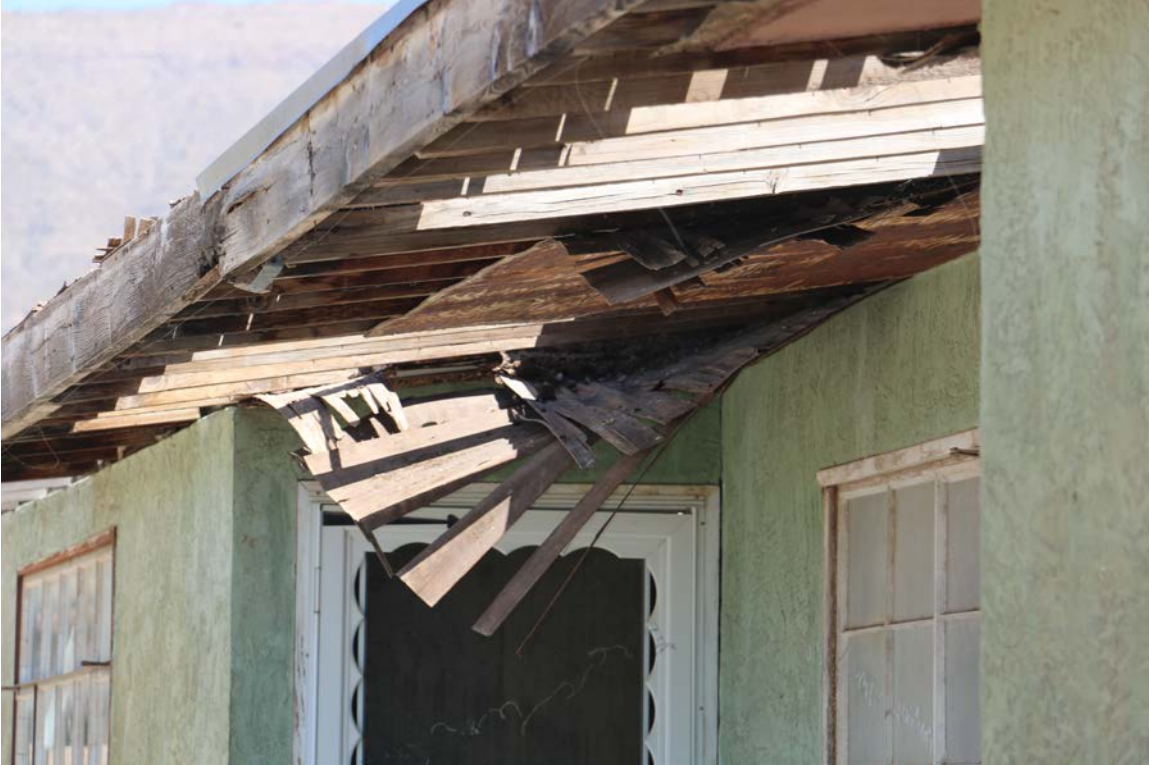
Photo # 18 front side
