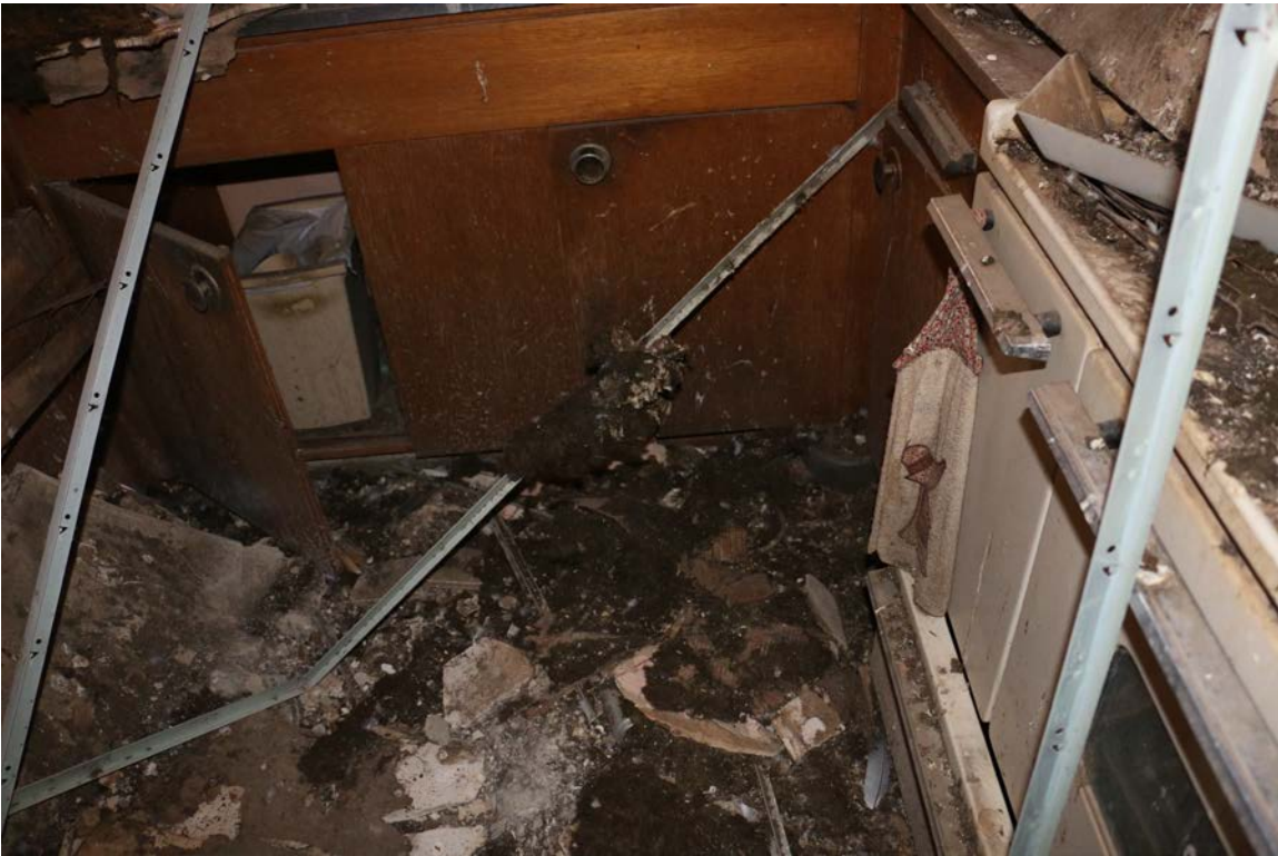
Photo #99 kitchen floor
