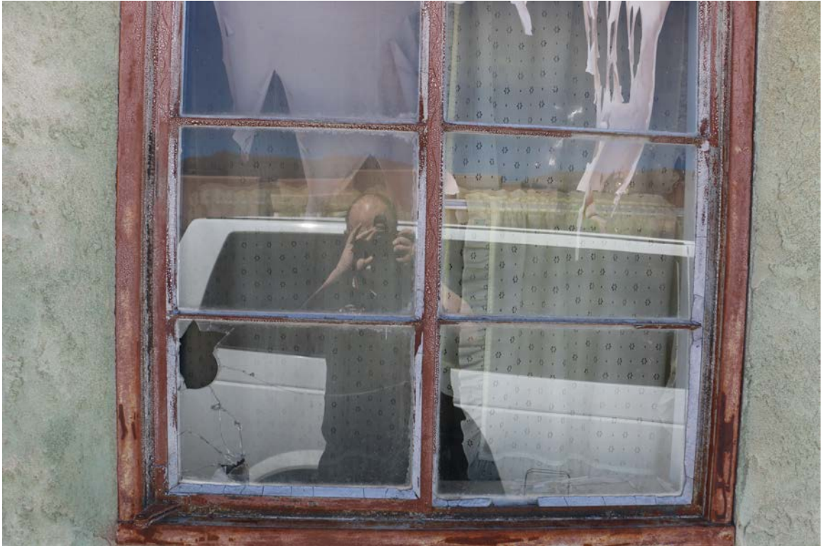
Photo #13 eastside window
