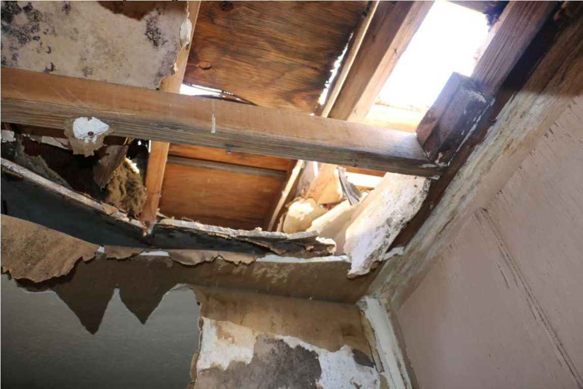
Photo #151 hallway ceiling to bathroom
