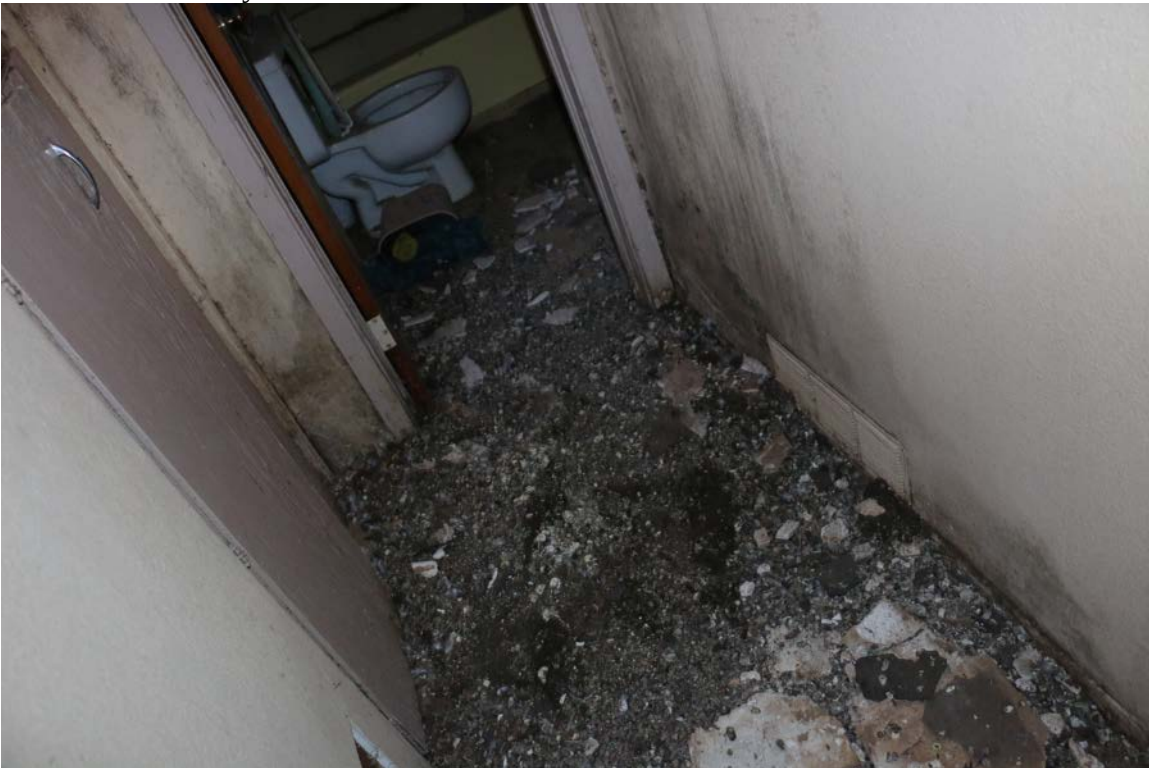
Photo #145 hallway to bathroom
