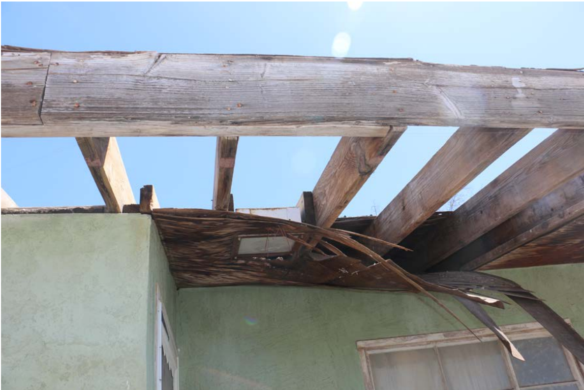
Photo #7 front side
