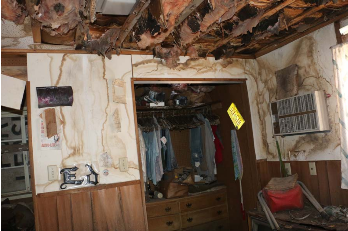
Photo #204 southeast corner room
