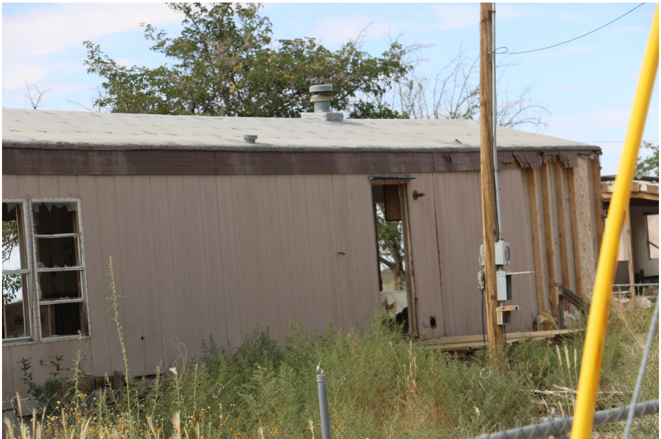
The backside of the trailer
