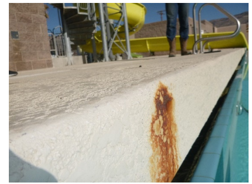
Exposed rebar/corrosion
