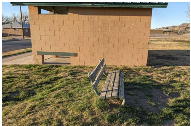
Restroom building and bench; turf grass is patchy.
