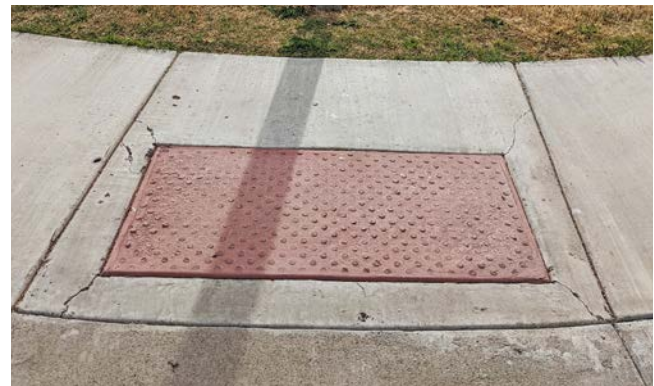
ADA ramp with truncated domes.
