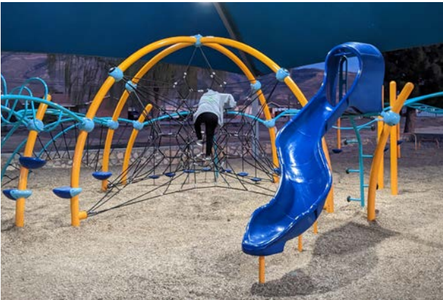
Play equipment with inadequate surfacing.
