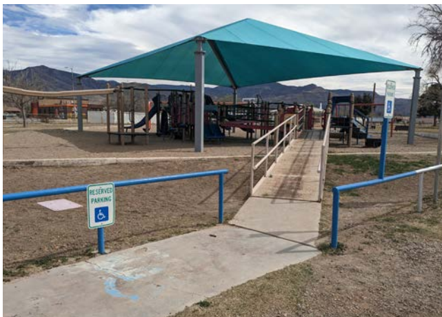
Accessible ramp leading to the playground.
