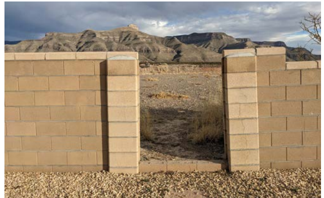
Unprotected access to gravel pit.
