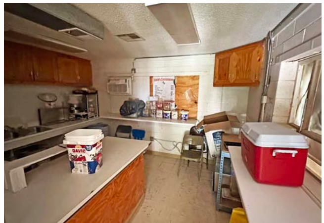
Press box concession building, first floor.
