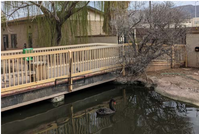
Pond needs new aeration and overhead netting.
