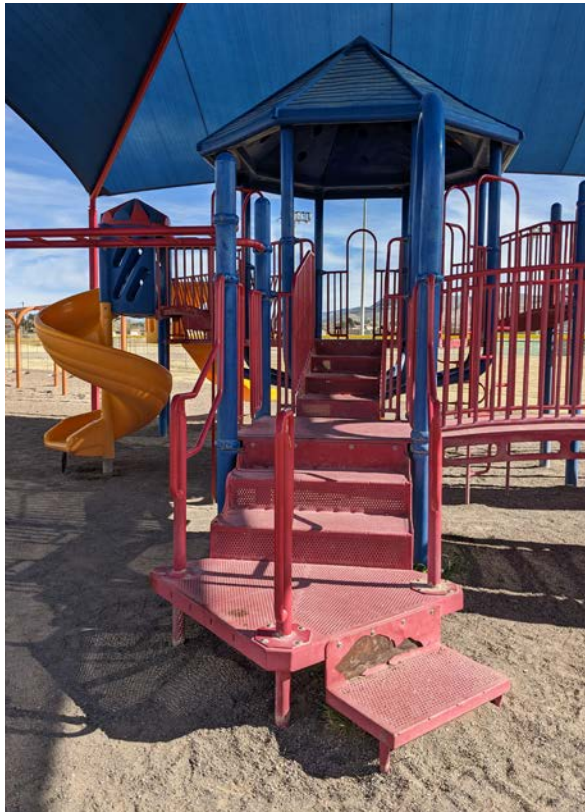
Playground equipment is showing signs of wear and tear.
