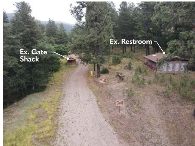
West Lake Campground entry.
