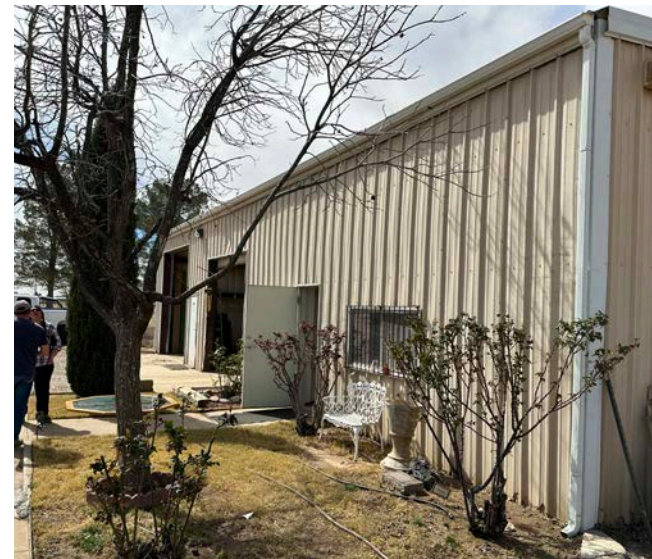
Existing maintenance and administration building exterior.
