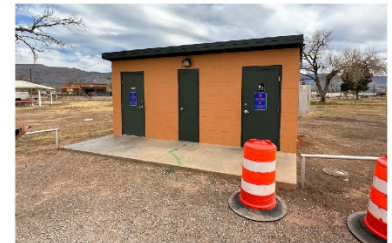
Typical restroom building at Alameda Park.
