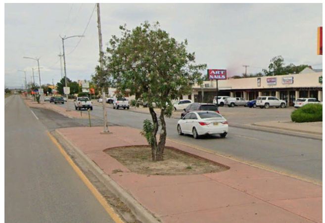
Median with stamped color concrete with cut out for the tree.
