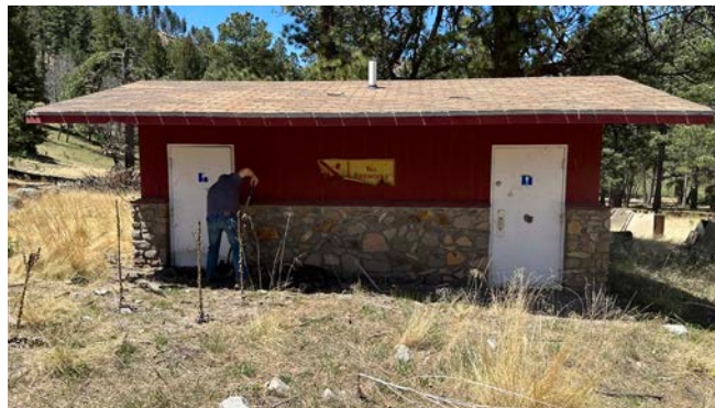
West restroom exterior at West Lake Campground.
