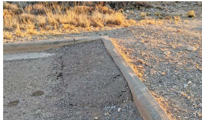
Informal asphalt ramp in the parking lot.
