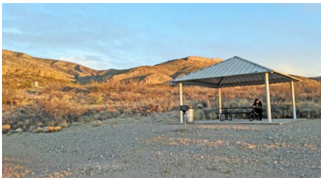
Shade structure and picnic table.
