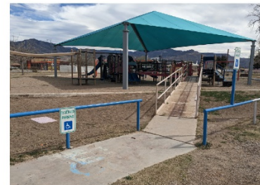
Accessible ramp leading to the playground.
