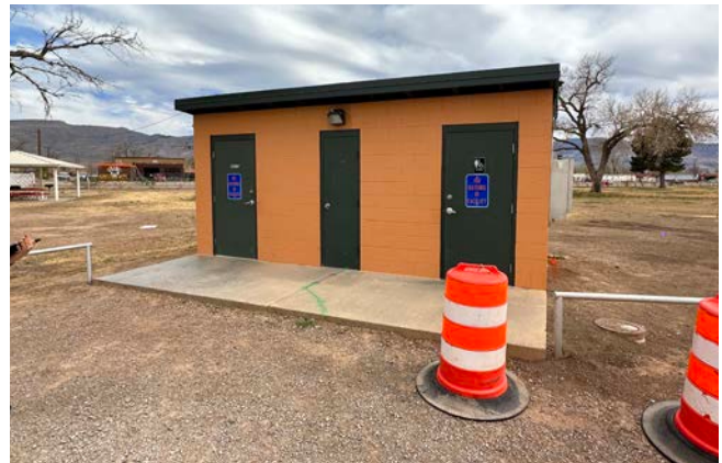
Typical restroom building at Alameda Park.
