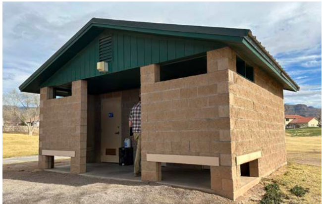
East restroom exterior.
