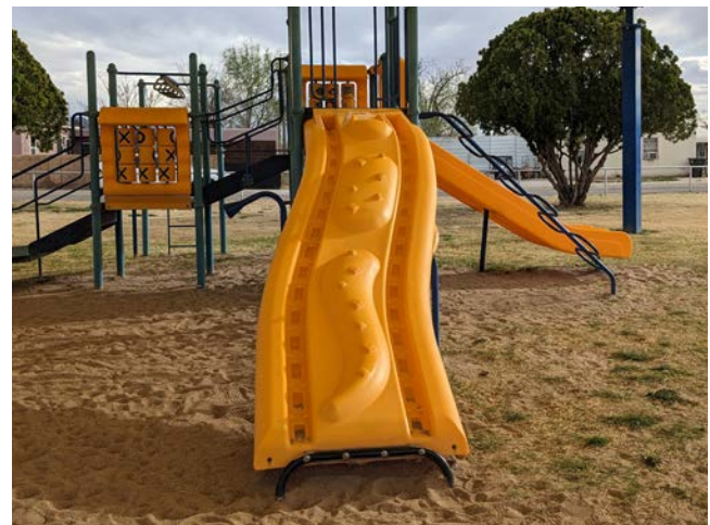
Inadequate playground surface with turf growing through it.
