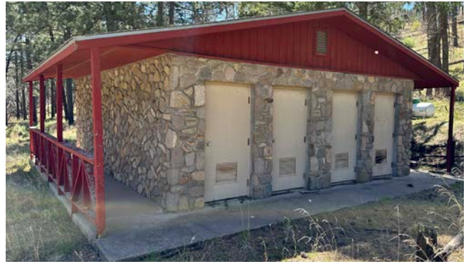
Restroom building at West Lake Campground.
