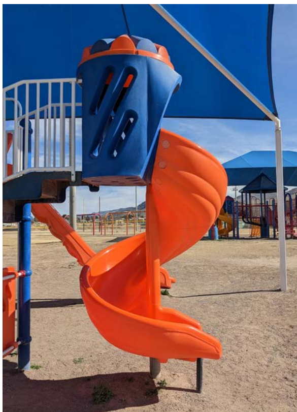
Lack of adequate playground surfacing.
