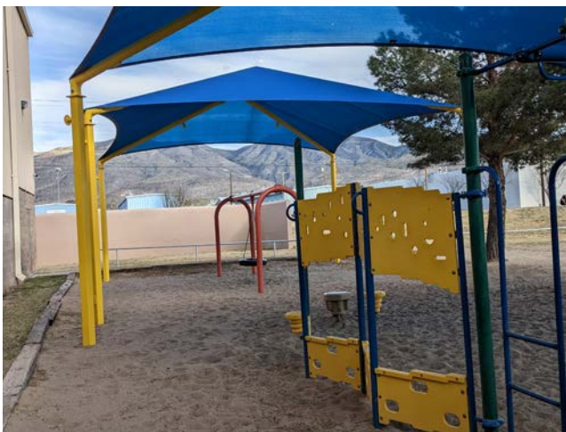
Drainage flows into the playground. Play area edge and surfacing are inadequate.
