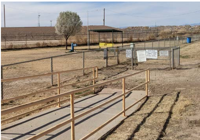
ADA access ramp and entry gate into Bark Park.
