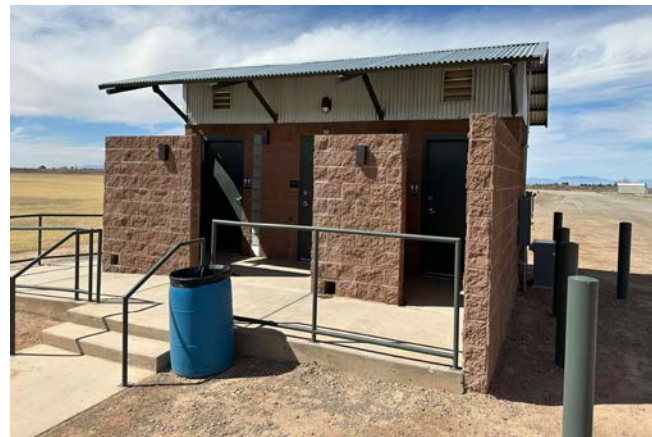
Recently constructed restroom.
