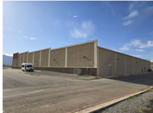
Looking southeast at the subject property
