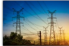
Micro Grids, Transformers, Frequency Regulation
